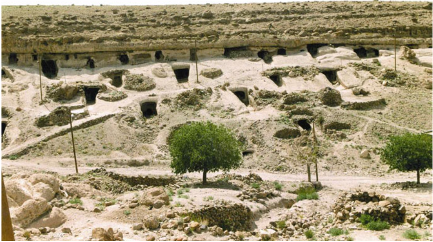
Fig. 1.3 Ancient rural dwellings in Meymand built in tuff and breccia and covered with hard agglomerate (northeast of Meydook)
