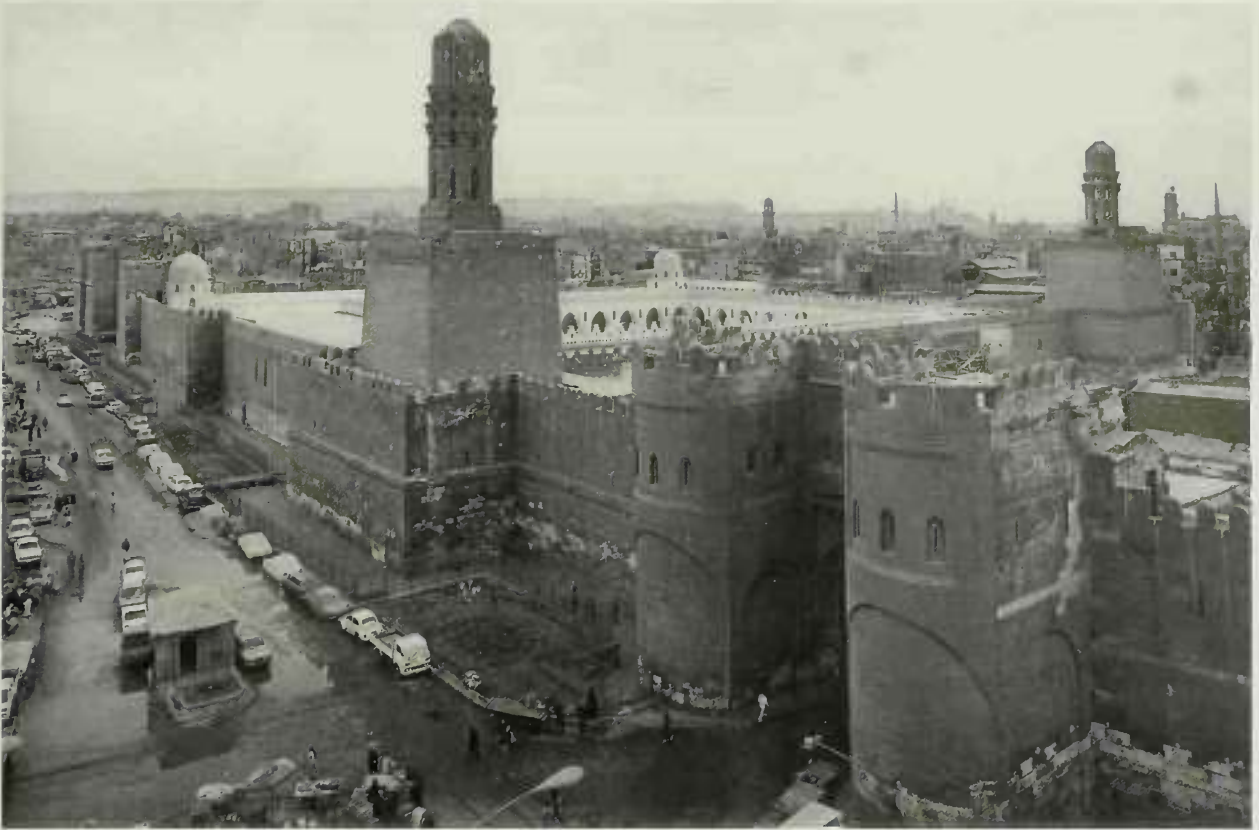
300. Cairo, al-Hakim Mosque, 990 and 1013, general view, and city walls, 1087
