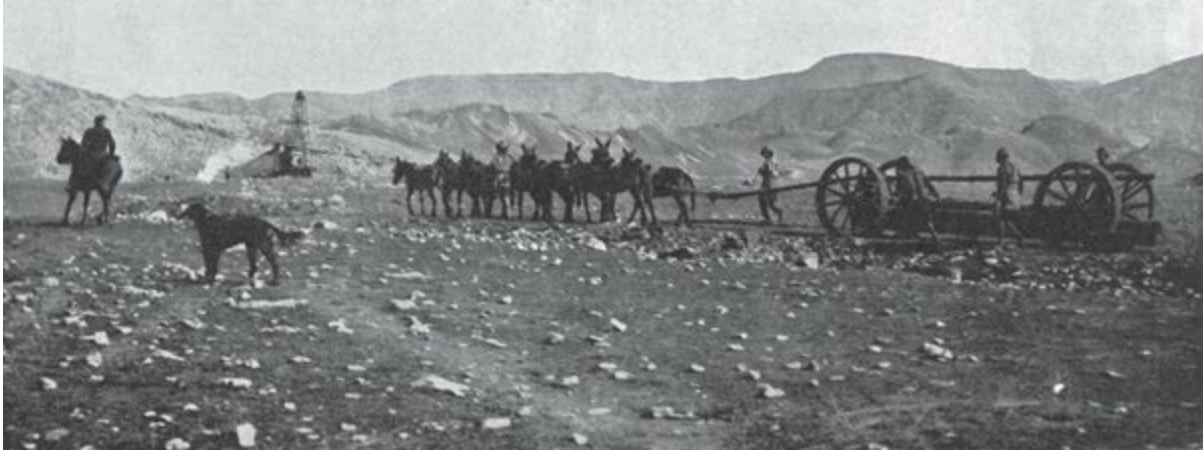
Figure 7.2. A section of casing for the Anglo-Persian Oil Company's pipeline being transported near Masjed Soleiman.
